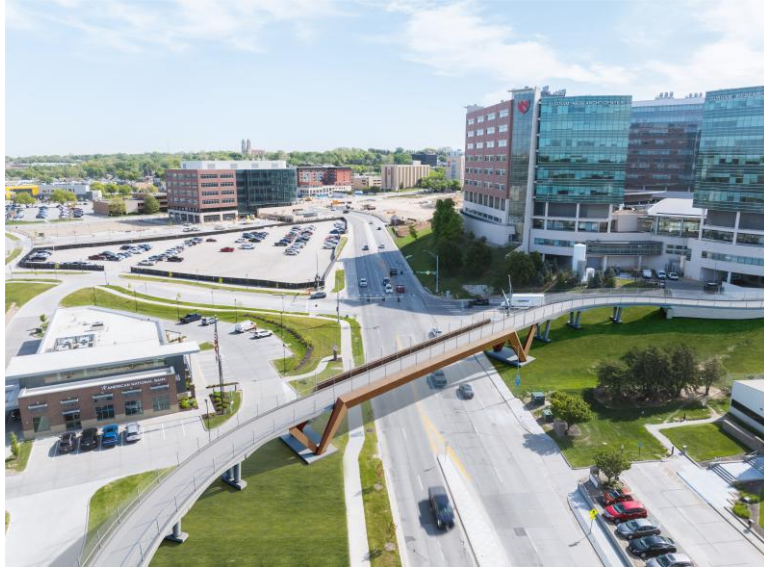
Saddle Creek Bridge at Emile Street
