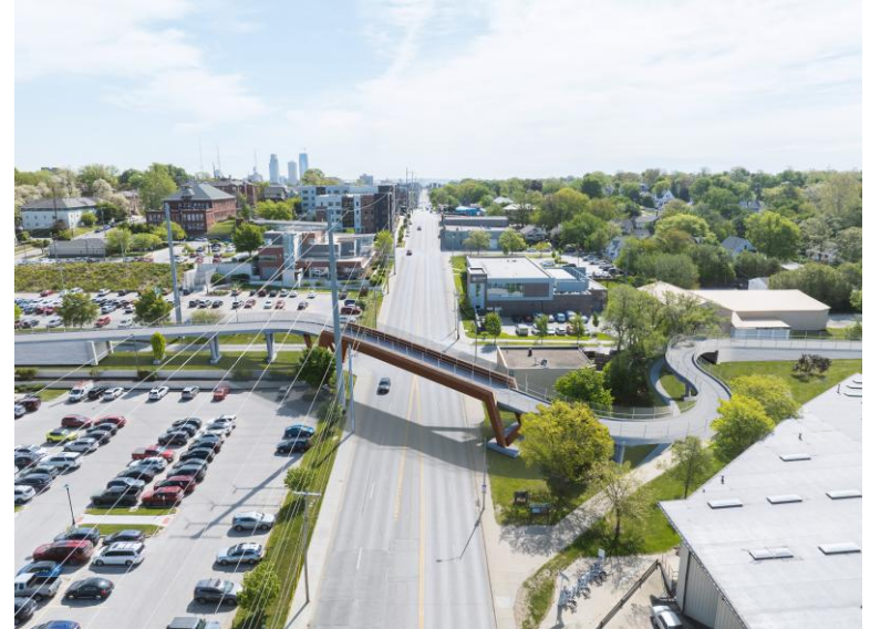
Leavenworth Bridge at 39th Street
